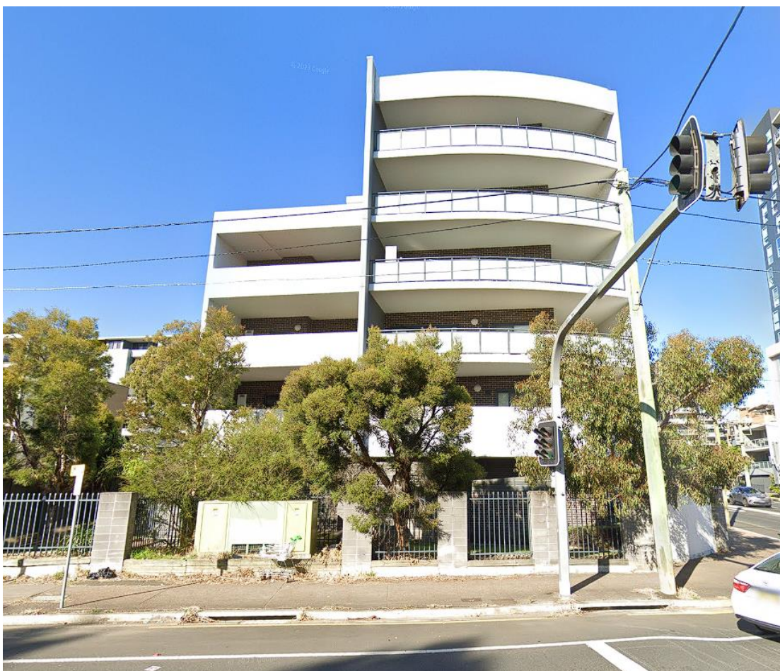
Figure 6: Existing 6 storey residential flat building on adjacent site to the west (Source – Google Maps 2023)
